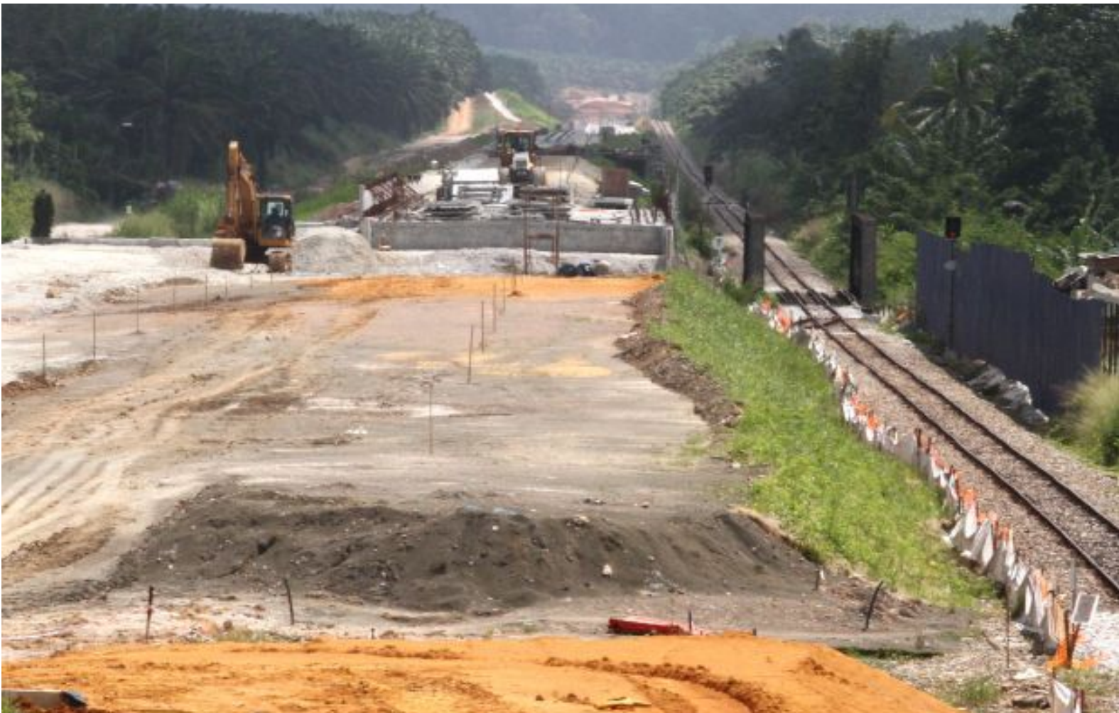
Double tracking rail construction near Gemas. - Filepic
